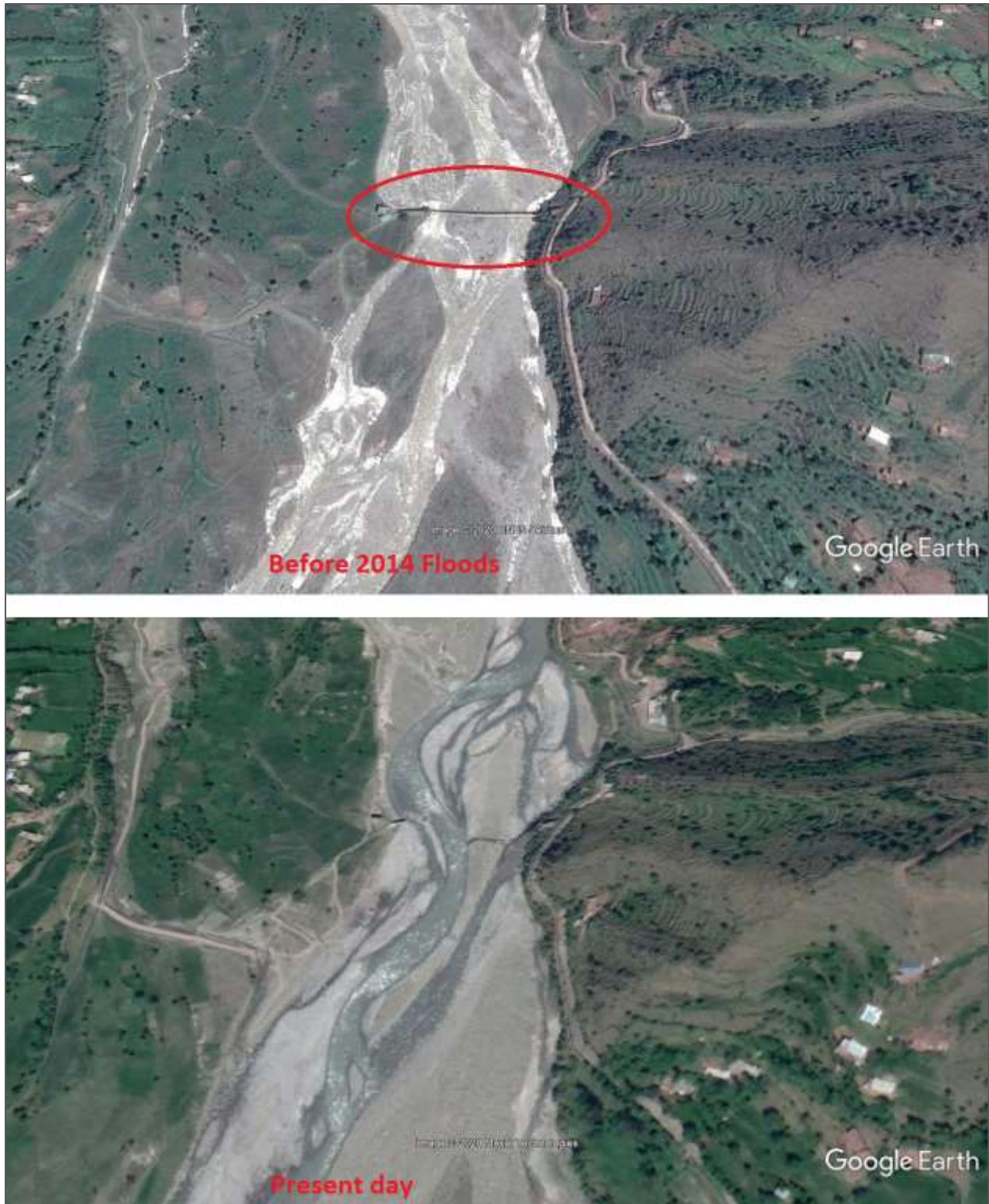
Figure 3.4: Bridge location before and after September 2014 floods
